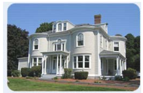
Glenhaven Academy, Marlborough, MA
